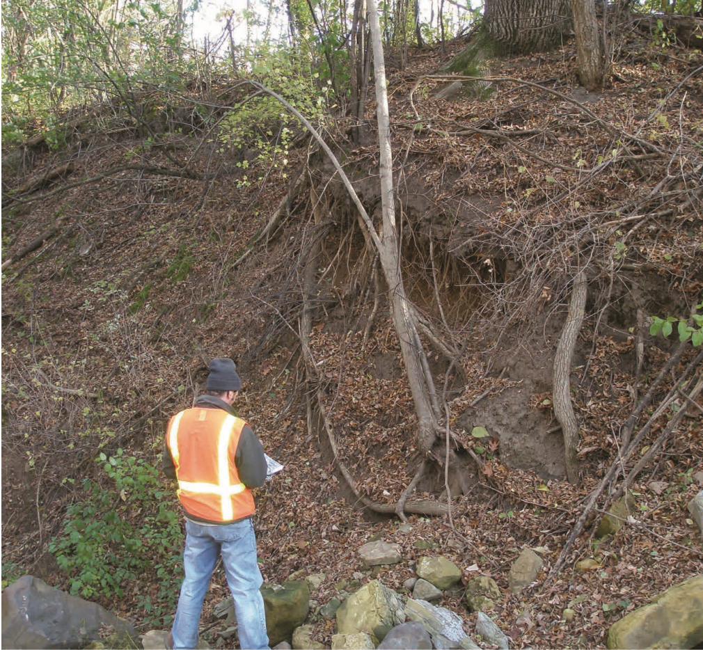
Erosion near the intersection of 30th St. and Trading Post Trail
